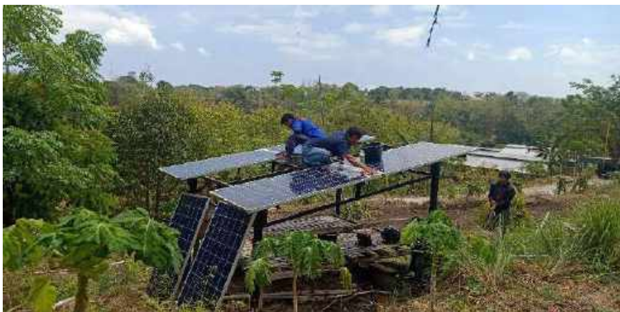
Gambar. Pembersihan panel surya
